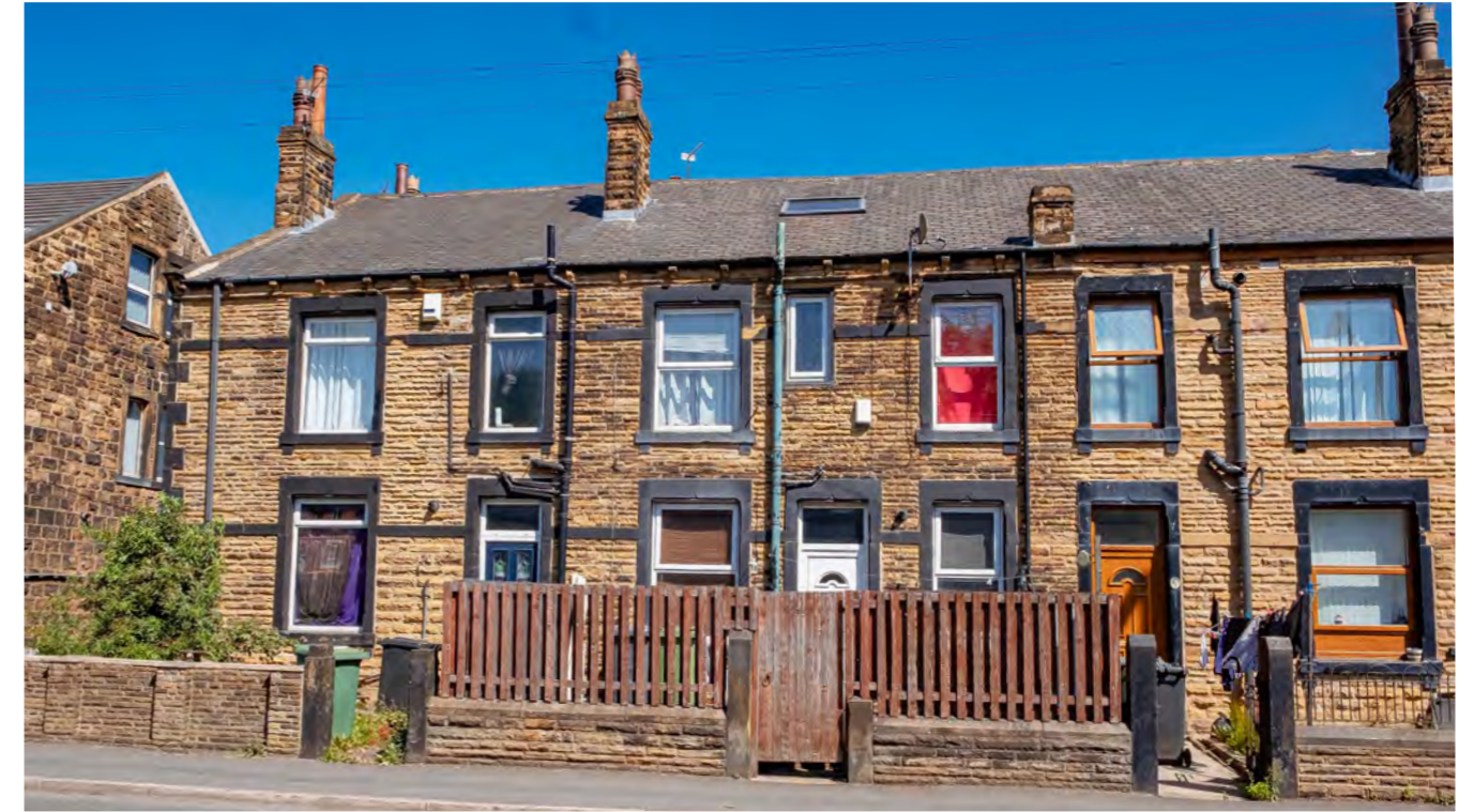
This area contains the distinctive mix of the industrial town; residential use intermixed with industrial activity and service provision including shops and places of worship. The regular grid-form of the settlement layout and the shared palette of materials unify the disparate architectural forms.
