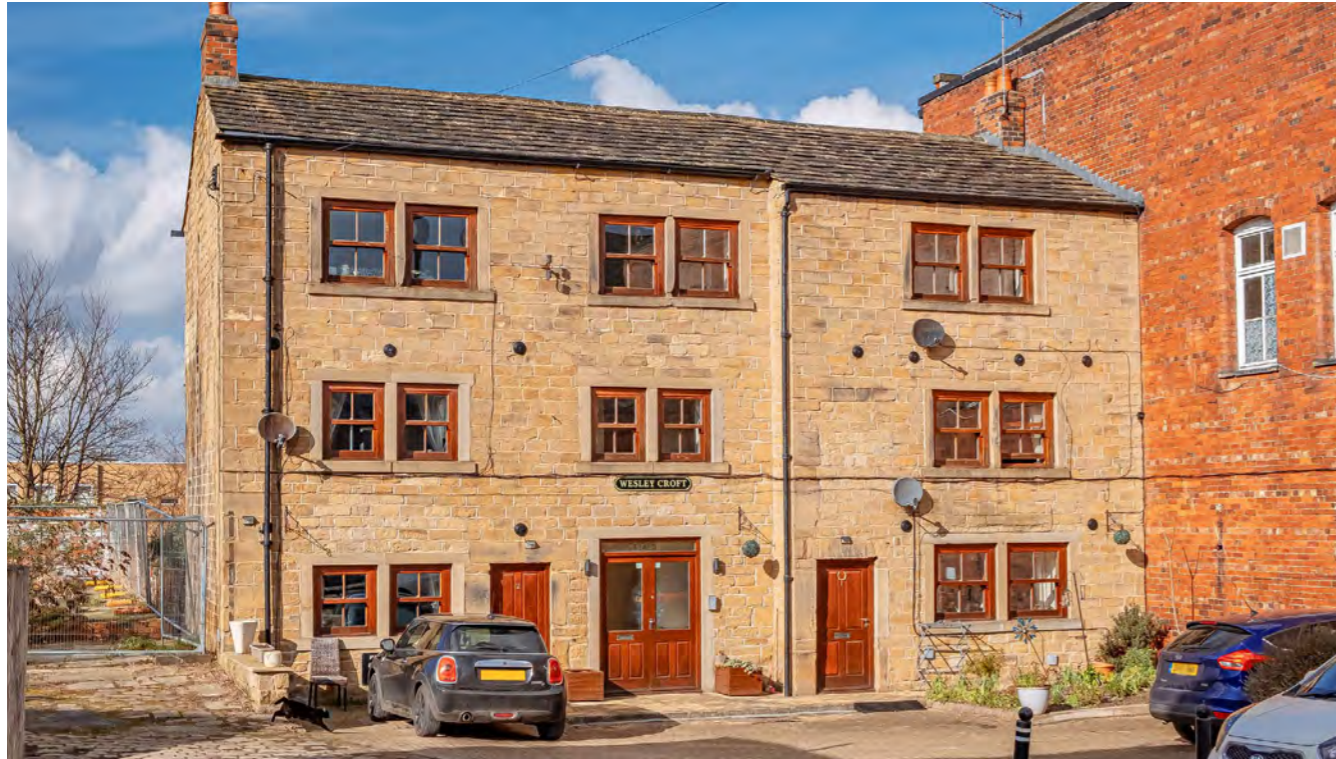
Above: 10 Wesley Street, grade II listed 18th century weavers cottage.
