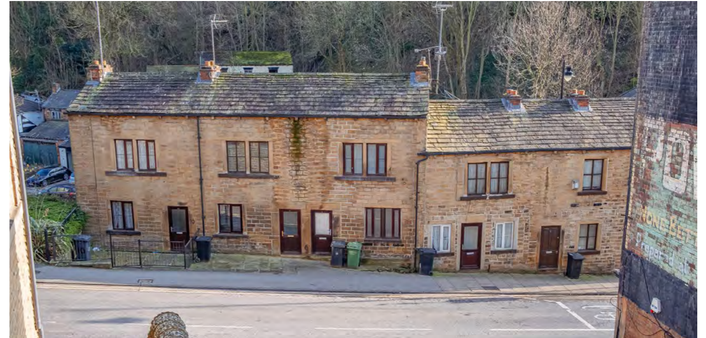
Below: Simply detailed 'double-decker' houses Chapel Hill, c1800, grade II listed
