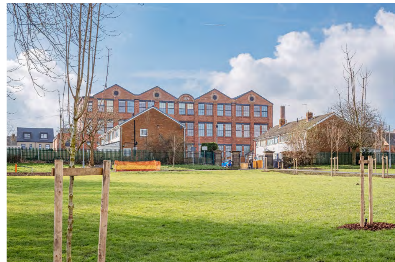
The area retains its industrial character with numerous important surviving mill complexes, including chimneys which act as local landmarks in the streetscape and skyline.
